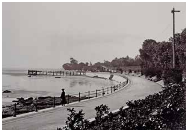
Promenade to Clare Lane pier before Lido construction
