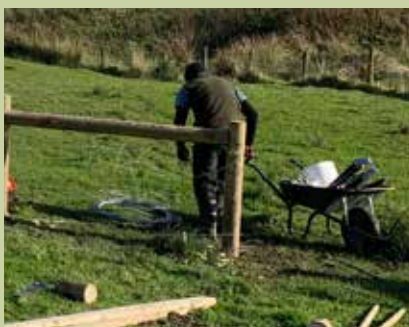
Volunteer from the Rivers Trust erect fencing
