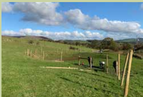
Fencing taking shape
