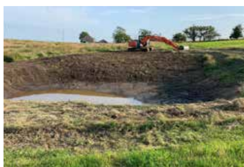
The pond is dug
